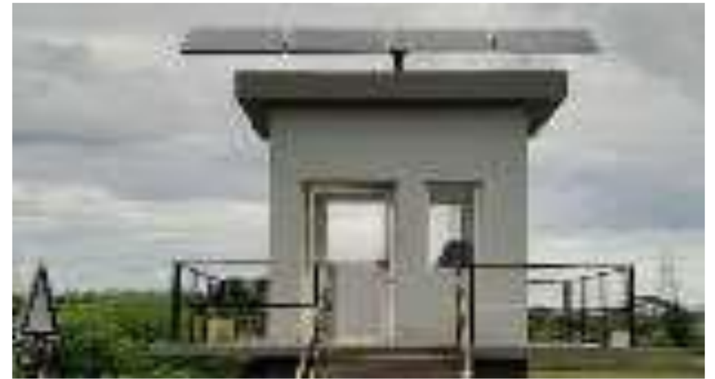
Solar panel at security post
